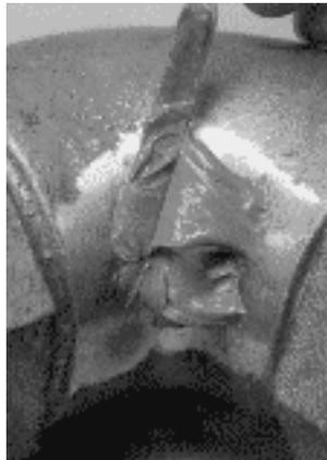
Press the backup plate in place, leaving a minimum thickness of at least 0.1 in (2.5 mm).
